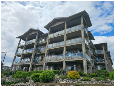
Before Picture showing the Left Side (South Side) of Building 1 Showing Wood Trim to be Painted
